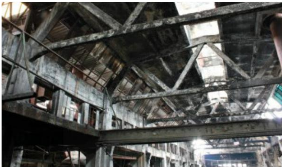
Picture 2. Main factory building roof construction
